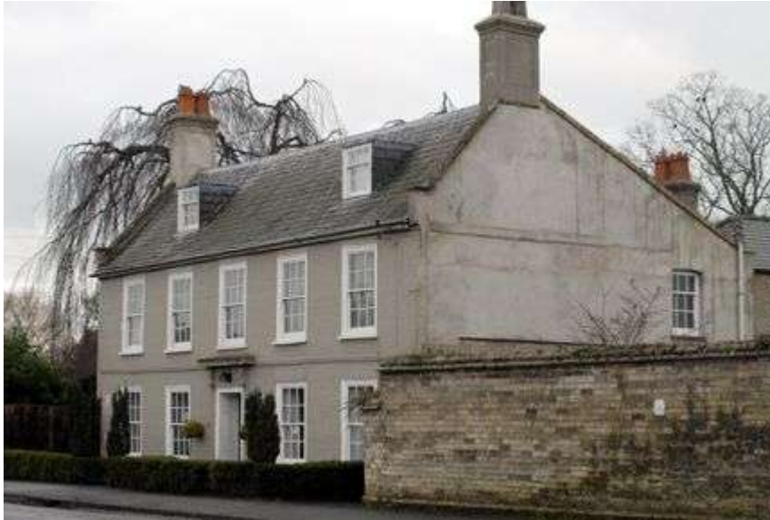
Addison House on Sand Street
